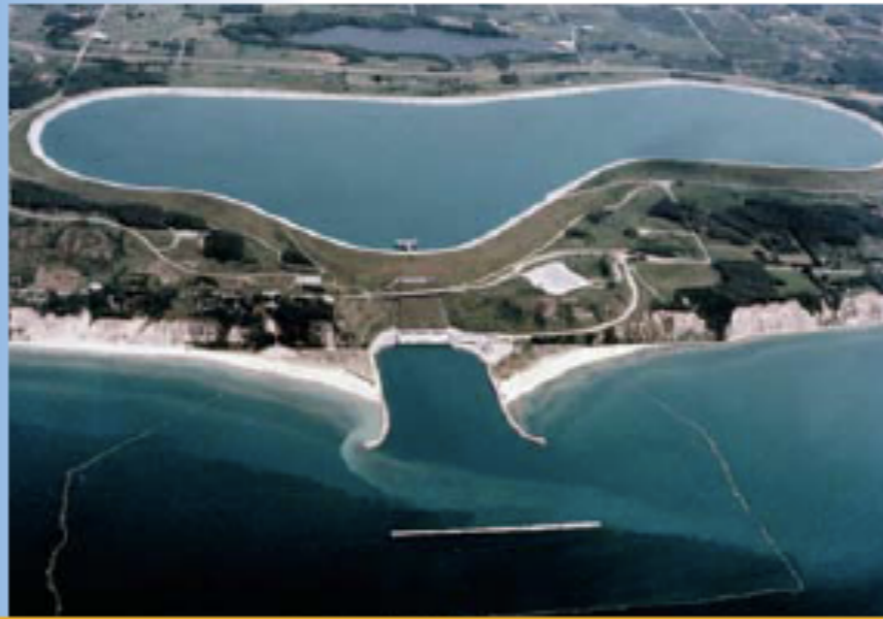
Ludington Pumped Storage has a capacity of 1,872 megawatts.
