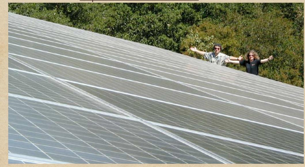
Adelmans' photovoltaic system. Santa Cruz CA!!! Our system has a 2,880 square foot array with a theoretical output of 30.5kW.
